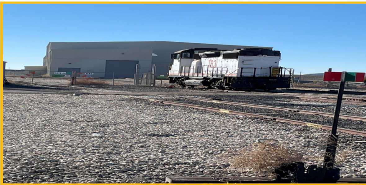
New construction East Side Rollover Facility (ESRF)
